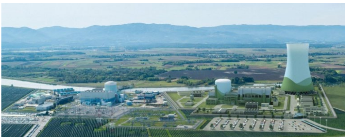
Figure 1: The location of the new JEK2 will be by the river Sava next to the existing Krško NPP (picture from website of GEN Energija, https://www.gen-energija.si/investiramo-in-razvijamo/drugi-blok-jedrskoelektarne-jek2- )
