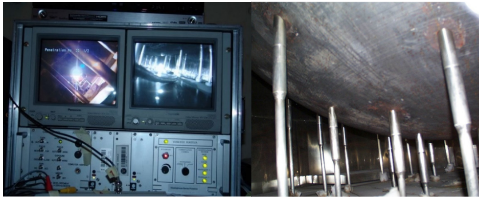
Figure 4: Visual inspection of penetrations on the RPV bottom
