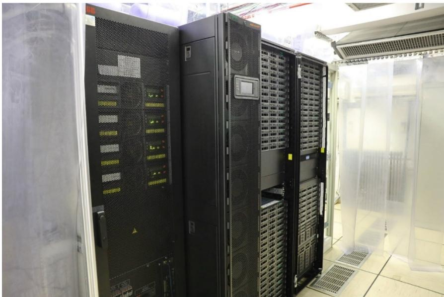
Figure 1: 80 kW modular UPS (left), (middle) 30 kW in-row cooling system and Skuta first two purchases (two racks on the right).
