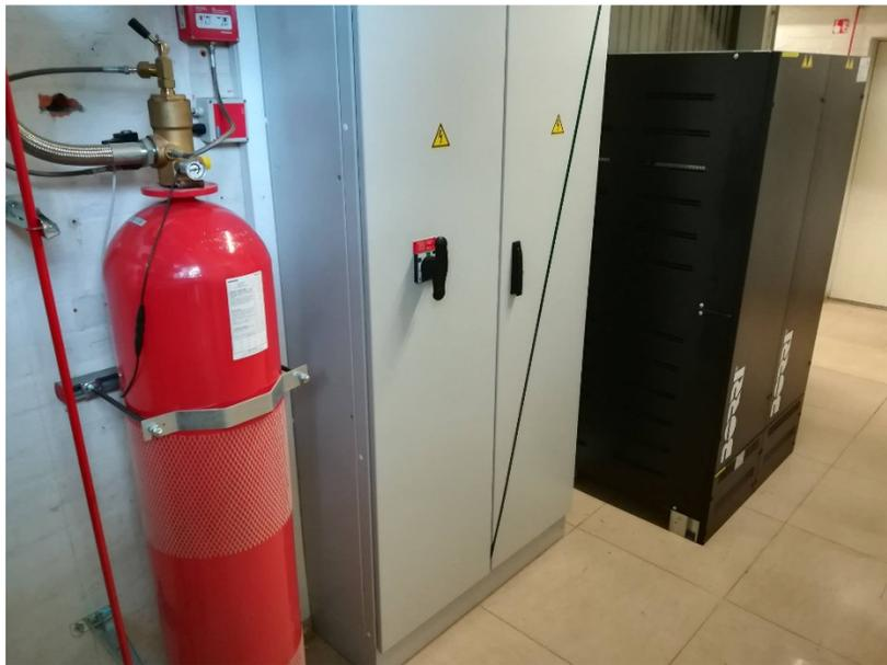
Figure 2: Flask of automatic fire protection system (left), new main electrical distribution board (middle), and (right) half of the modular UPS system – rack of lead batteries providing several minutes of power for entire cluster.
