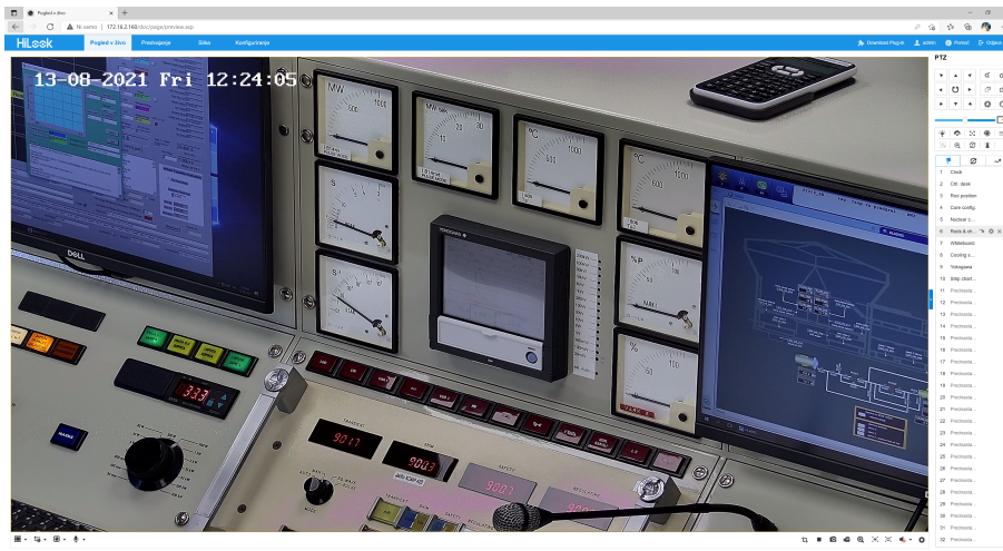
Figure 4: Dome camera pointed to the nuclear instrumentation. It could be remotely moved and zoomed-in to any point in the control room by using controls on the top right corner. Predefined positions (such as instrumentation and rod positions) could be selected in the table on the right side of the image.
