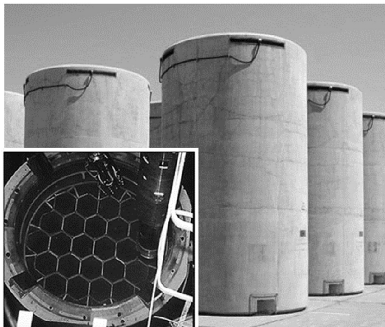
Figure 1. VSC-24 dry storage container [8]
